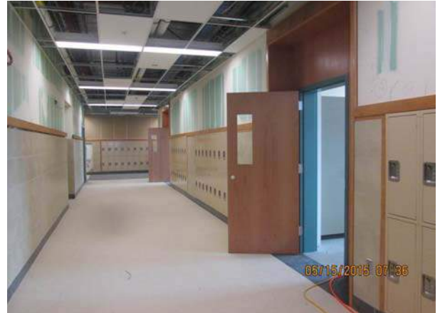
Building A - LPS: Lockers & Classroom Doors
