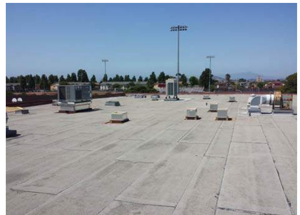
Roof Curbs & HVAC Units
