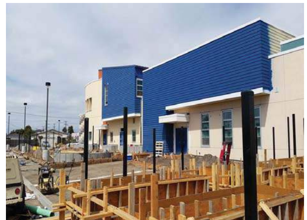
Building A Hardscape
