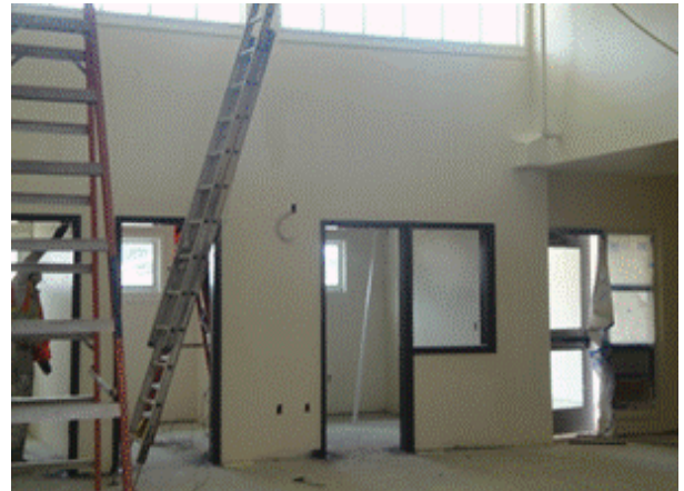
Building D - Sheetrock of walls
