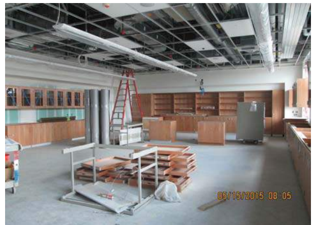
Building C - Science Classroom Casework
