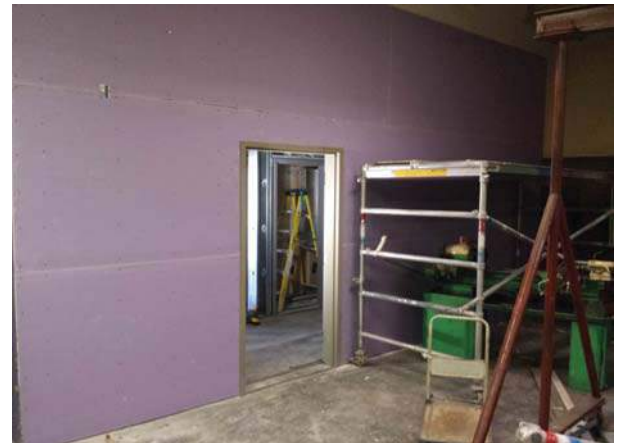
Interior Gypsum Board Wall
