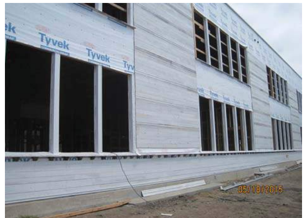
North Building Wood Siding
