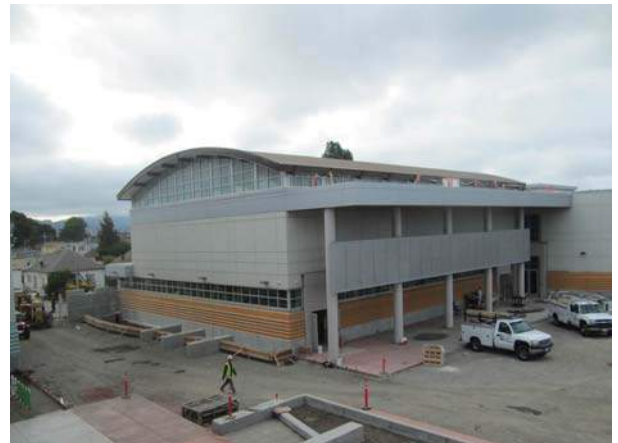
Site - Courtyard view from LPS
