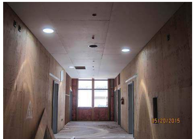
Gypsum Board at Corridor Ceiling
