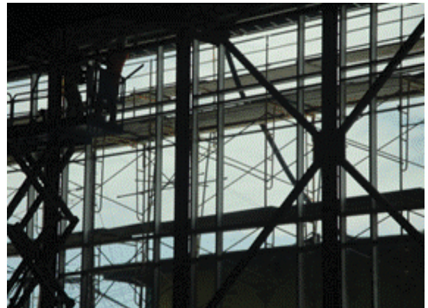
Building B - Window Installation in Gym Area
