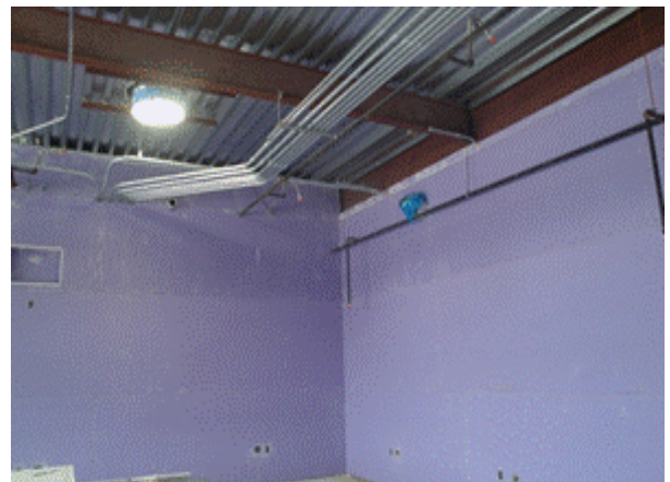
Duct Rough in and Electrical Wire Pulling
