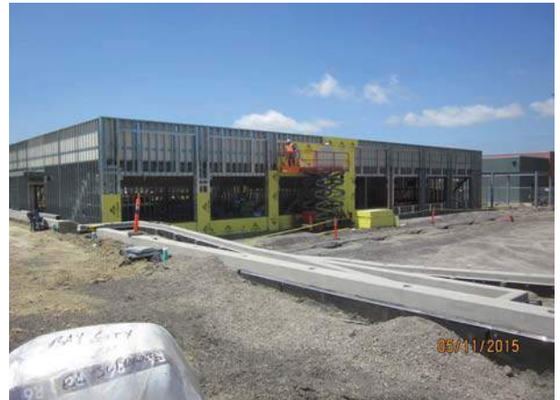
Exterior Wall Framing
