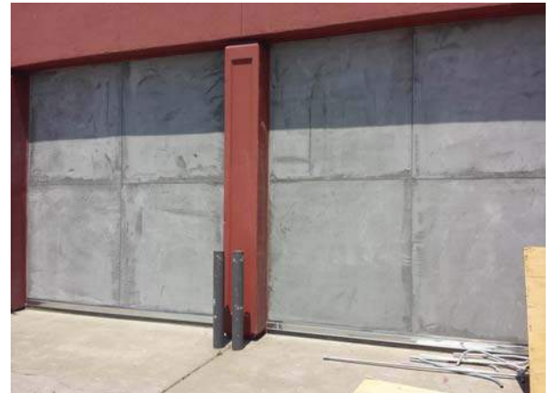
Exterior Stucco Coat
