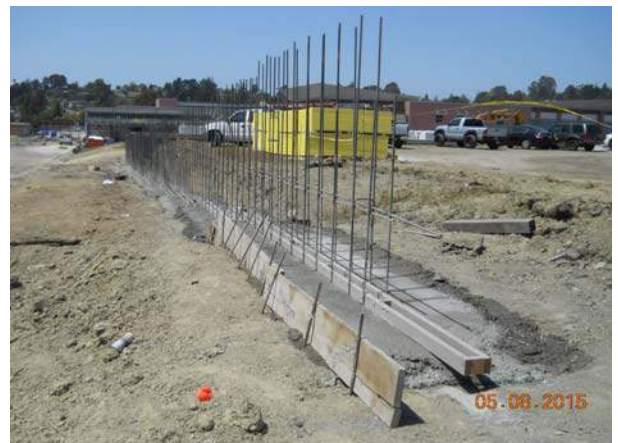
Retaining Wall Re-Bar
